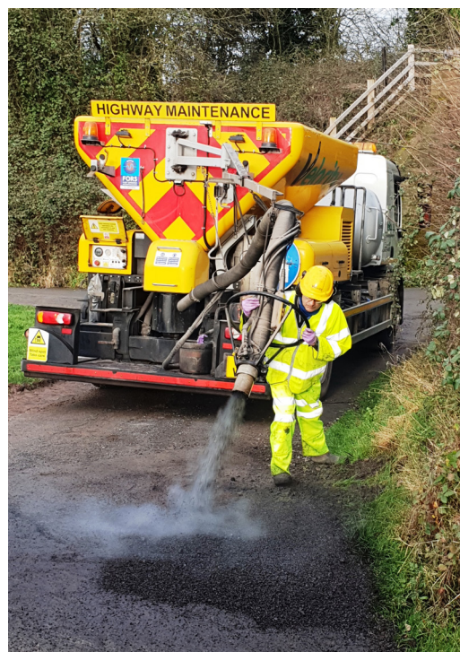
Road patching using Velocity's system
